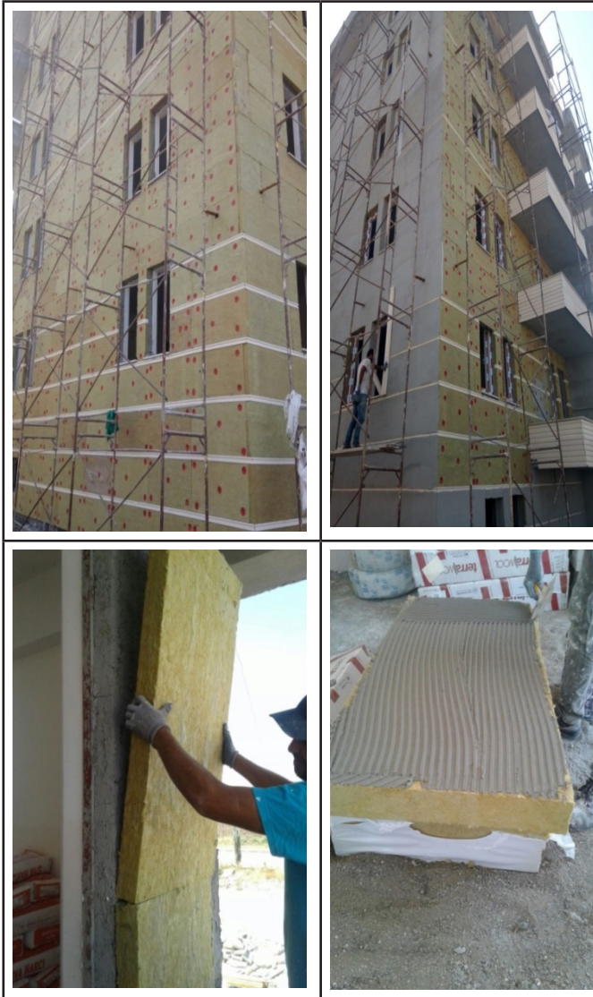
Figure 1. External Heat Insulation (Sheathing)
